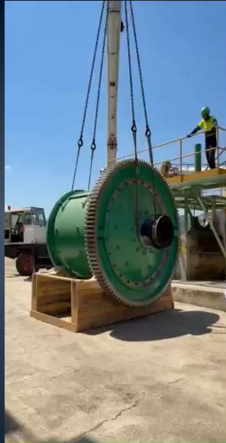
Mill lifting & positioning
